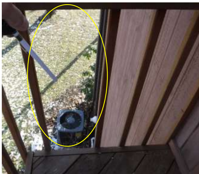
Figure 1 Recommend a carpenter evaluate balcony and make repairs; missing baluster/dangerous/safety hazard.
