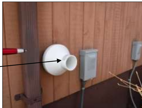
Figure 11 Recommend a vent screen PVC exhaust/vent for the furnace to keep out animals, etc.
